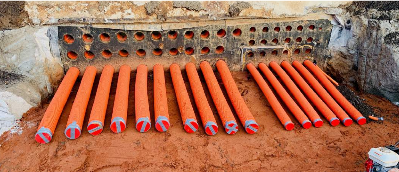
HPFLEX® Corrugated Joiner Ø100 & Ø150
